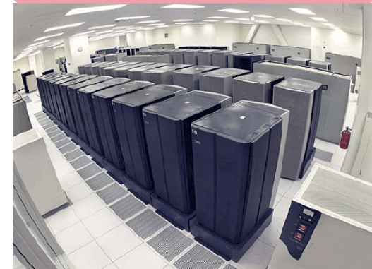
Converged Data Center
